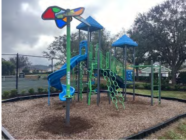
Playground equipment overview
