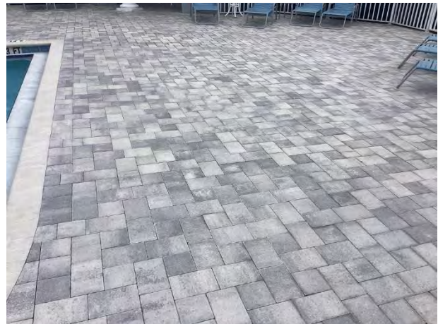
Paver pool deck overview
