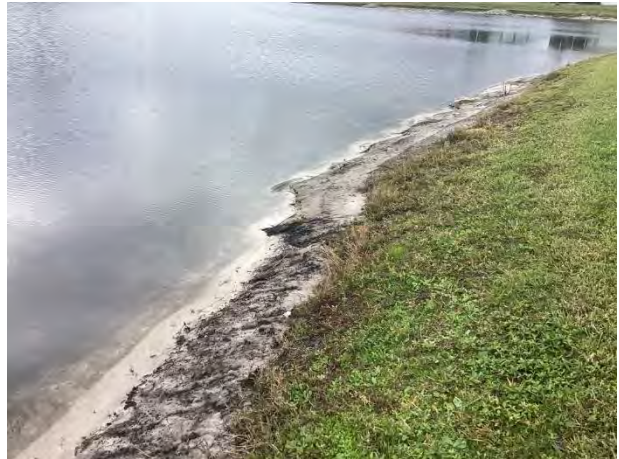
Previous shoreline repair Pond P
