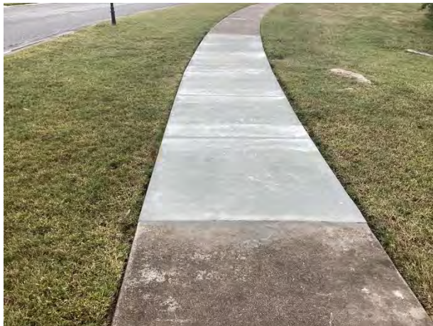
Concrete sidewalk repair
