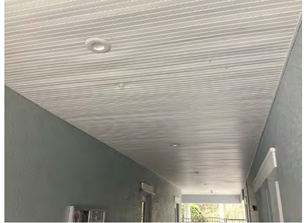
Vinyl soffit overview
