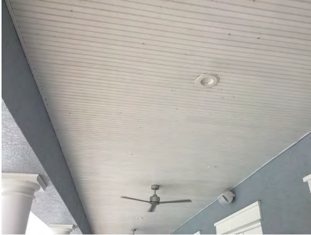
Vinyl soffit overview
