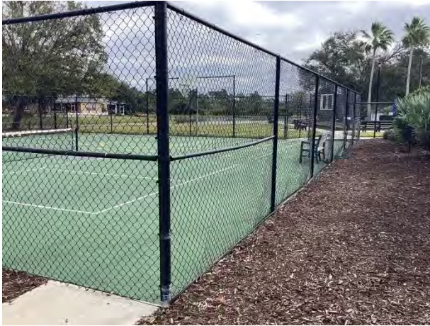
Chain link fence overview
