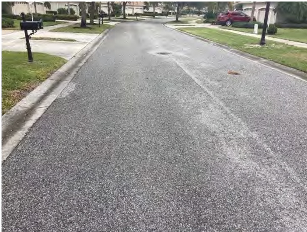
Pavement overview - Scarlet Avenue
