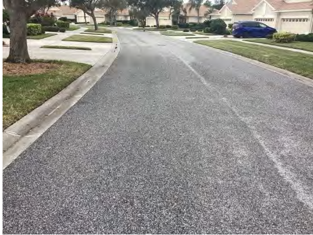
Pavement overview – Magnolia Circle
