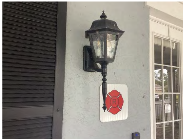
Exterior light fixture
