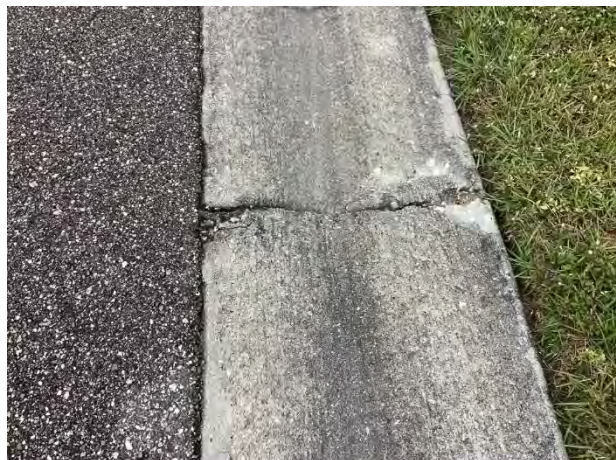
Concrete spalls
