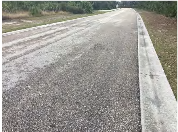
Pavement overview – Sycamore Drive
