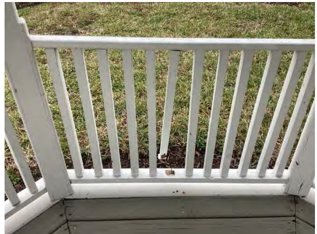
Damaged picket
