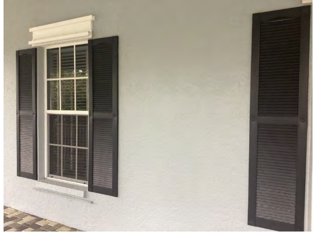
Stucco wall finishes
