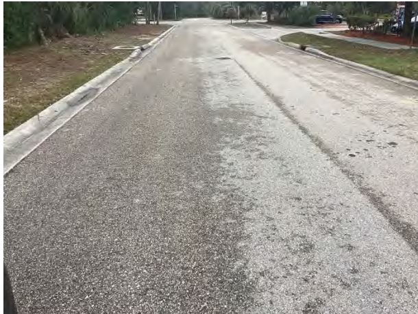
Pavement overview – Sycamore Drive
