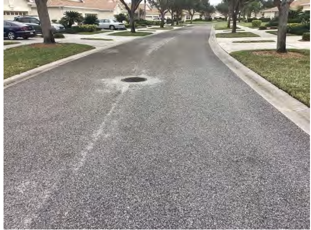
Pavement overview – Magnolia Circle
