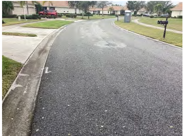
Pavement overview - Scarlet Avenue
