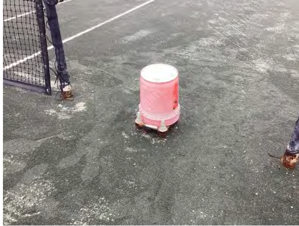
Light pole and fixture base
