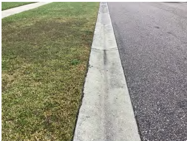
Concrete curb and gutter
