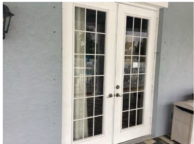
Common windows and doors
