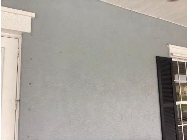
Stucco wall finishes
