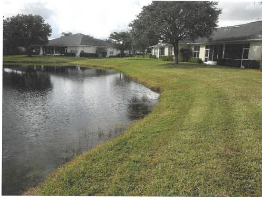
Figure 4: Lake 8 – Erosion along the northwest bank.
