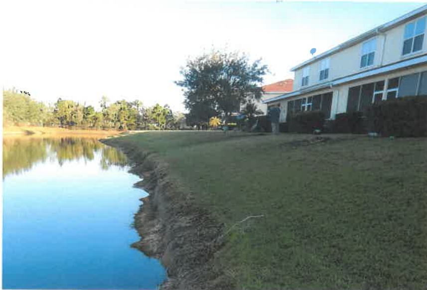
Figure 14: Lake 19 - Facing north along east bank.
