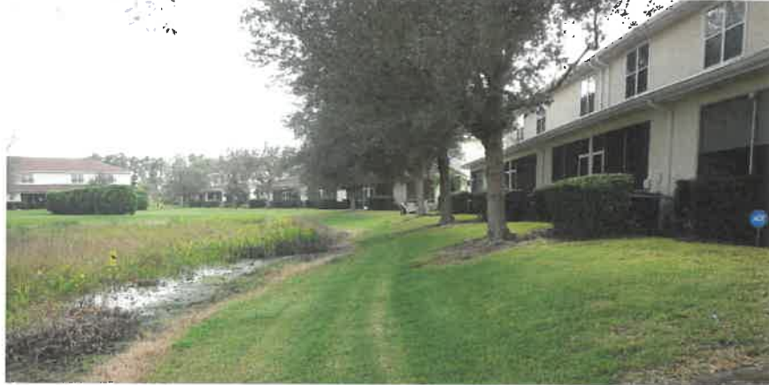
Figure 13: Lake 17 - Erosion and steepening banks at south end of townhomes.
