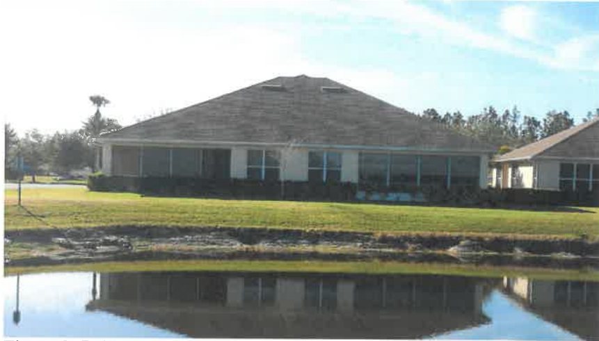
Figure 2: Lake 7 - Erosion along the south and east bank.
