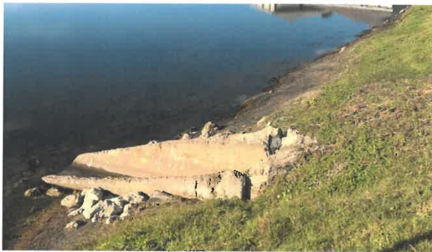
Figure 7: Lake 11 - Exposed mitered end.
