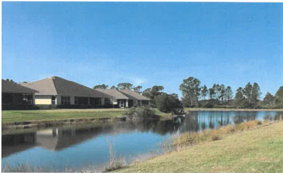
Figure 1: Lake 7, Photo 1, facing south bank where steep bank slope has formed
