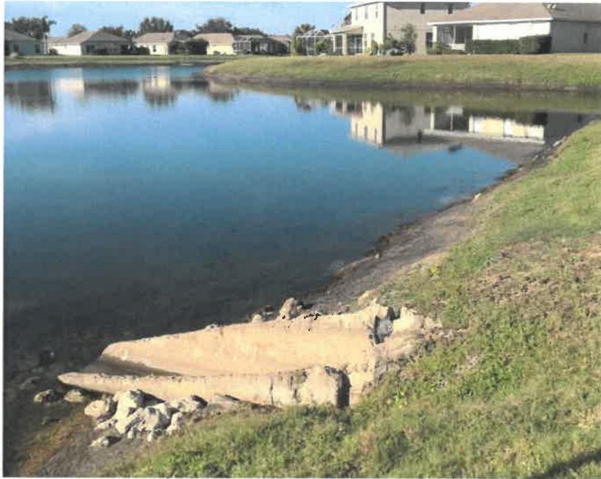
Figure 5: Lake 11, Photo 16, repair rip-rap/add new around exposed pipe
