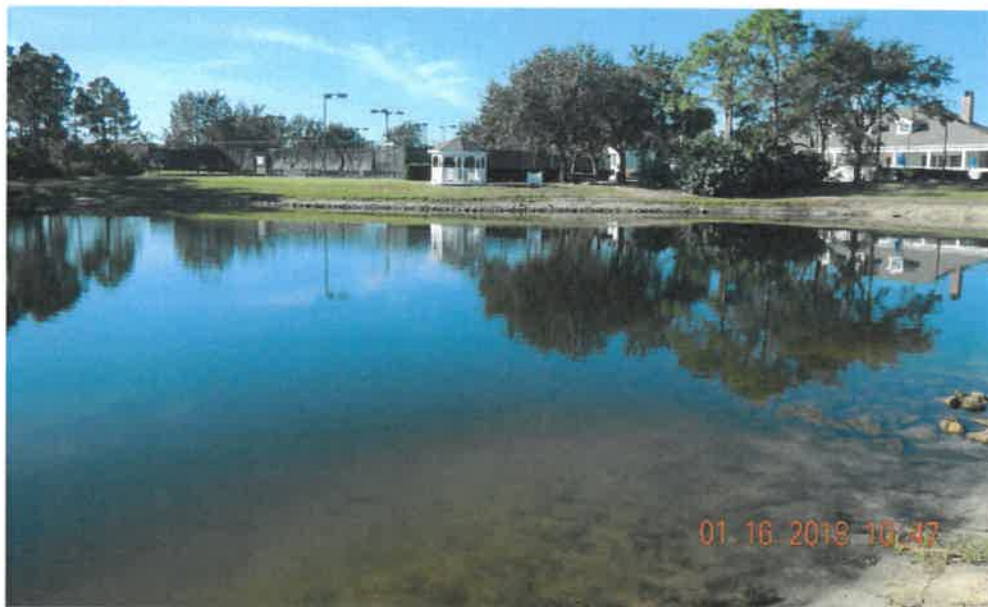
Figure 3: Lake 10, facing Southeast where bank is stabilized
