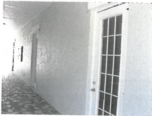
Stucco facade at clubhouse
