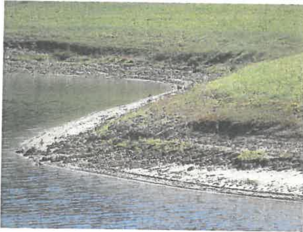
Pond B - shoreline erosion
