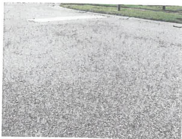
Typical condition of asphalt pavement
