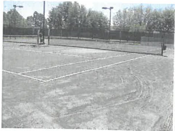
Tennis court overview
