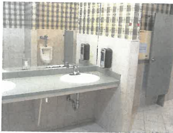
Rest room finishes and fixtures
