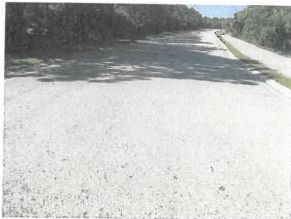
Asphalt pavement overview at Sycamore Street
