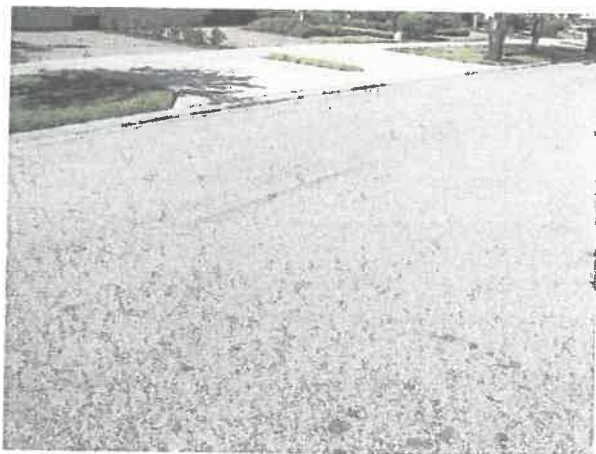
Asphalt pavement at Scarlett Avenue
