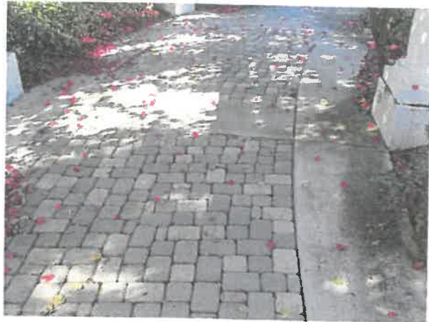
Pavers at community entrance
