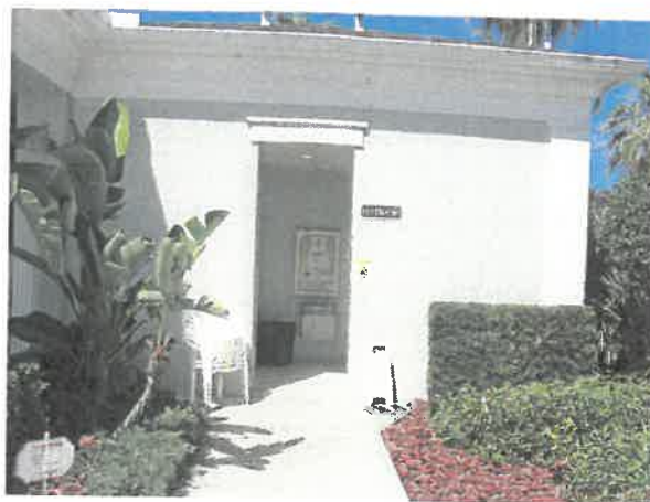
Stucco facade at clubhouse
