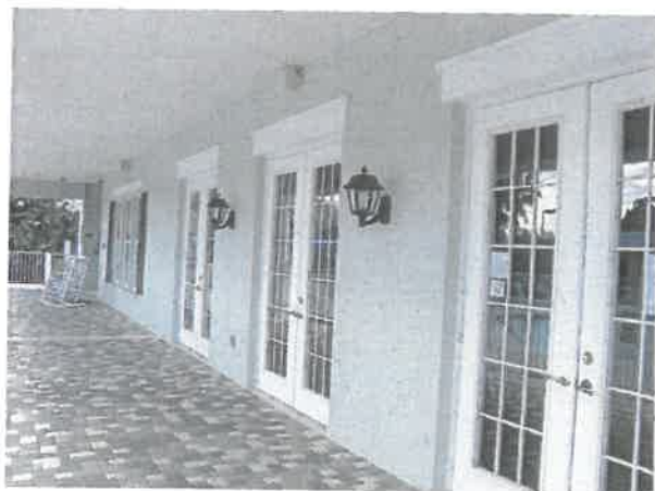
Stucco facade at clubhouse
