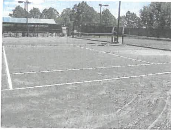
Tennis court overview
