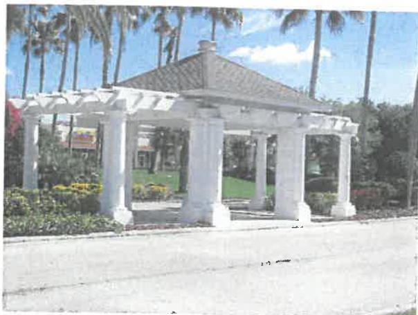
Entrance feature roof
