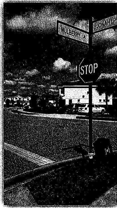
Figure 2: 24”x24” Stop Sign with Faded Reflectivity
