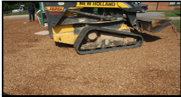
Use a track loader to speed compaction in larger areas.
