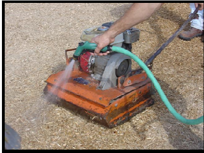
Use a compactor in small areas
