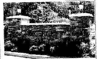
(B) Solid Monument, Stone Facade on Concrete Block Core
