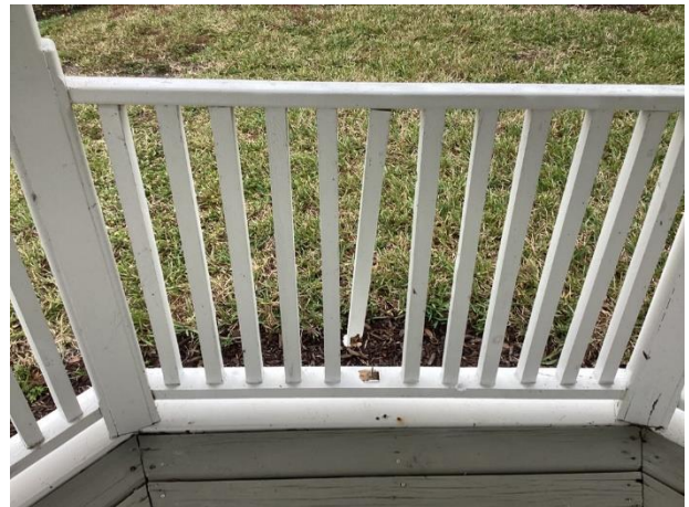
Damaged picket
