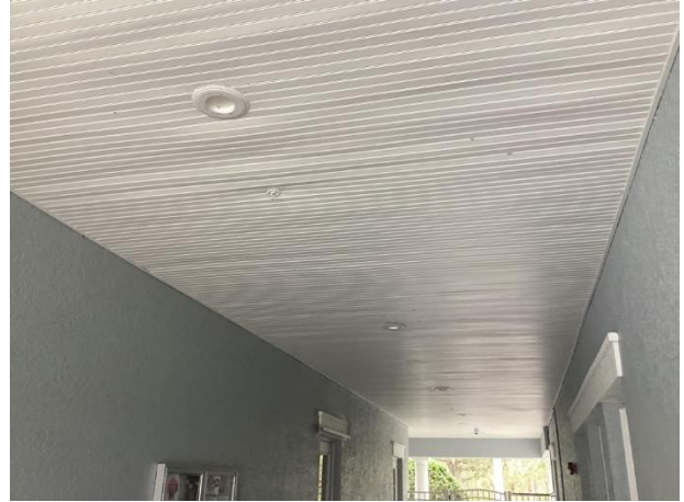
Vinyl soffit overview
