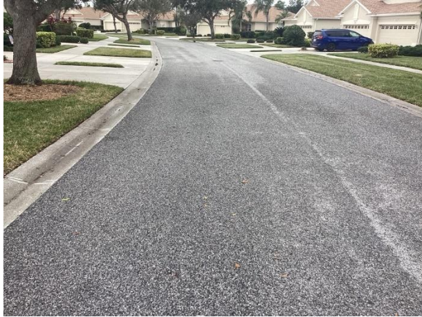
Pavement overview – Magnolia Circle
