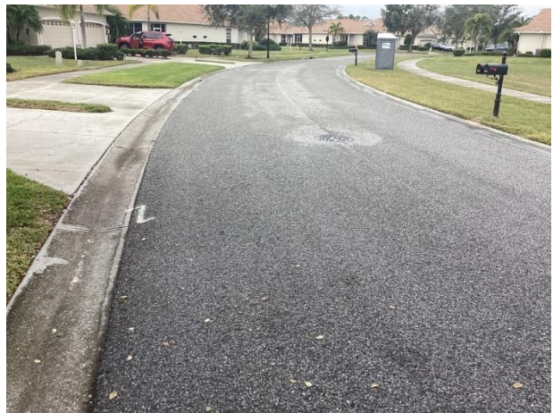
Pavement overview - Scarlet Avenue
