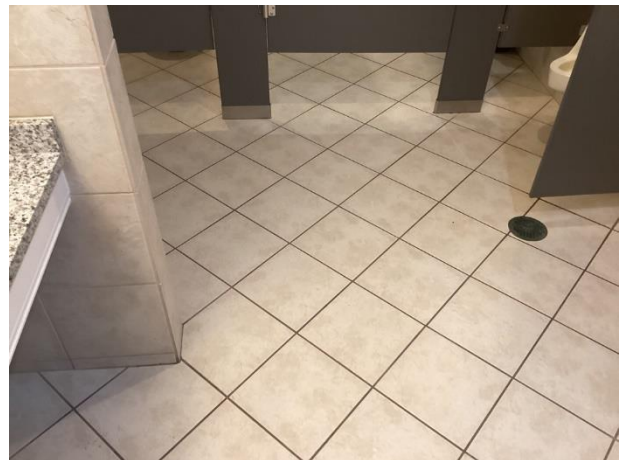
Rest room overview
