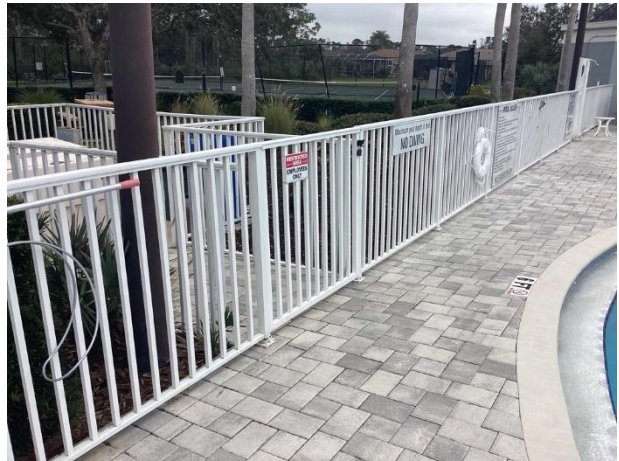
Aluminum fence overview
