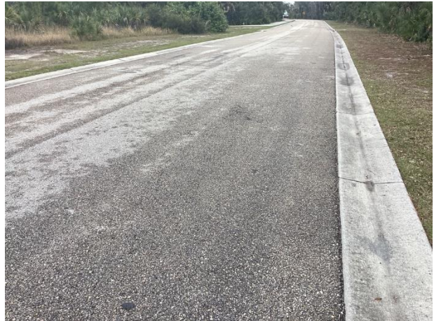
Pavement overview – Sycamore Drive
