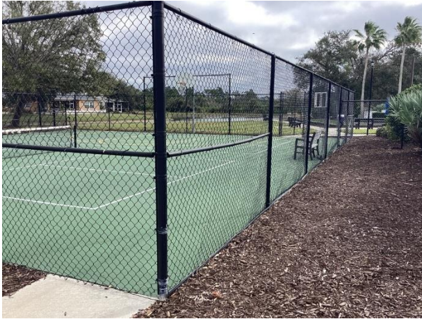
Chain link fence overview
