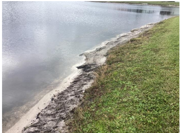
Previous shoreline repair Pond P
