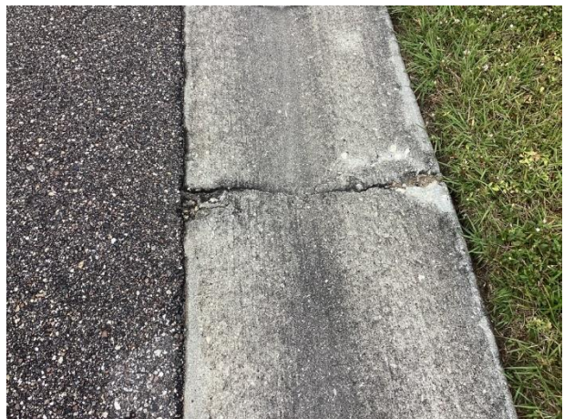
Concrete spalls
