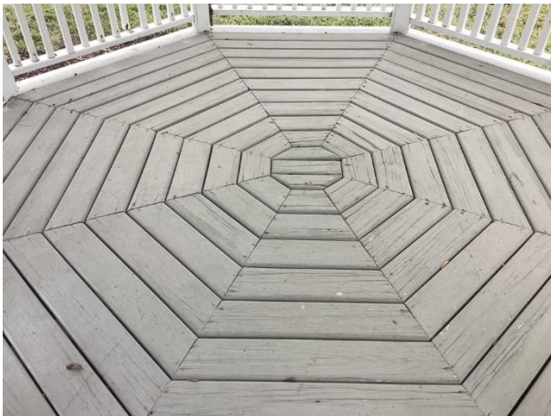
Wood deterioration
