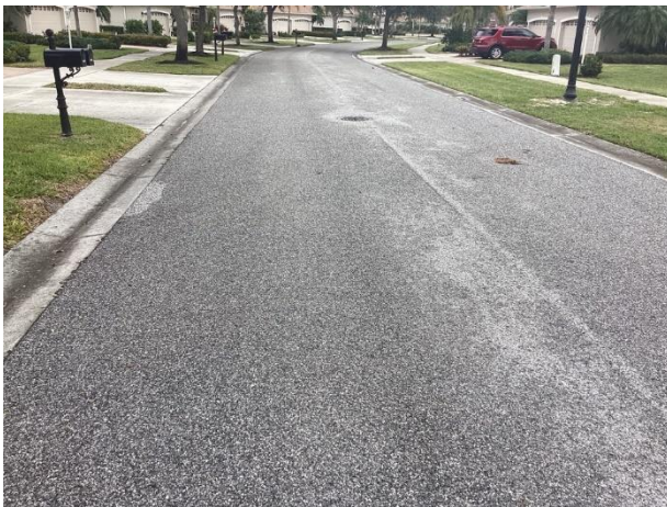
Pavement overview - Scarlet Avenue
