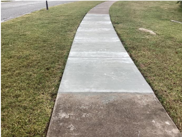
Concrete sidewalk repair
