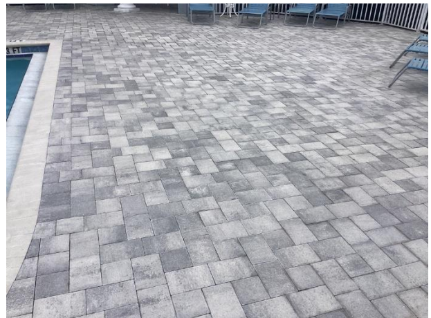
Paver pool deck overview
