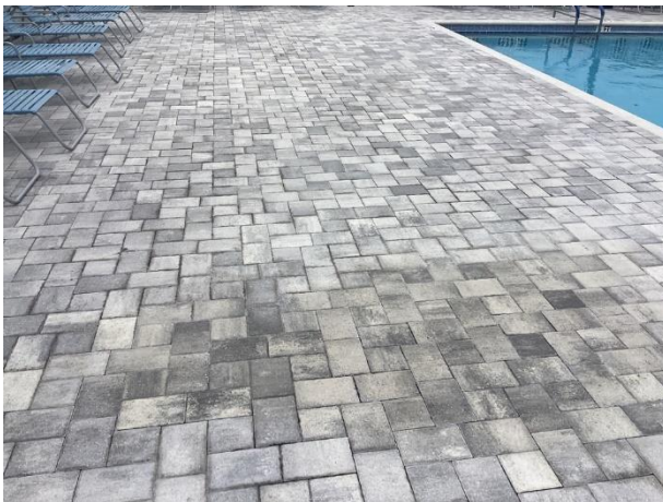
Paver pool deck overview
