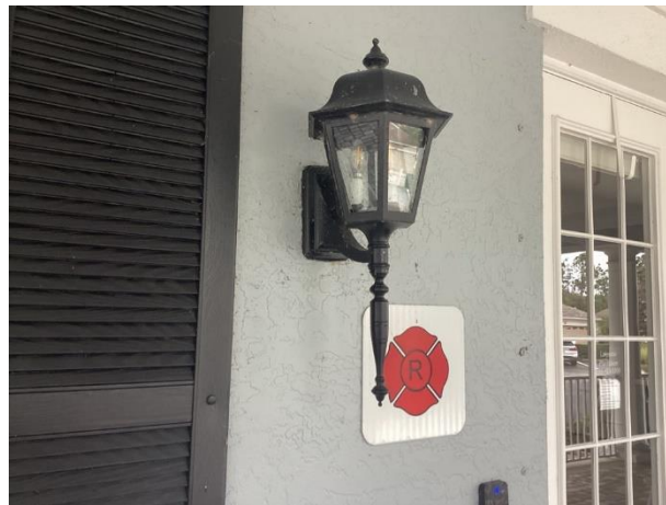
Exterior light fixture
