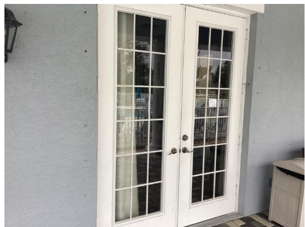
Common windows and doors
