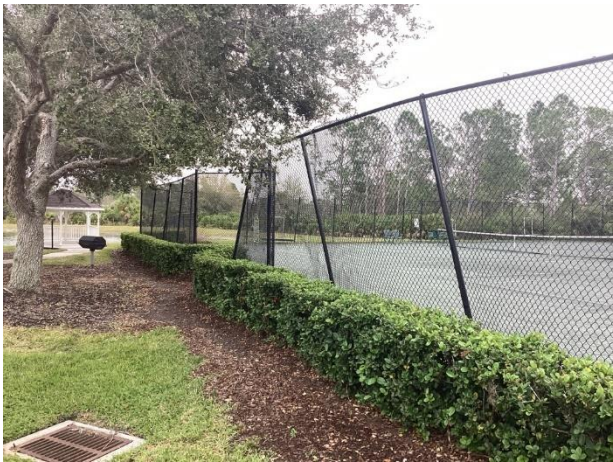
Fence leaning section
