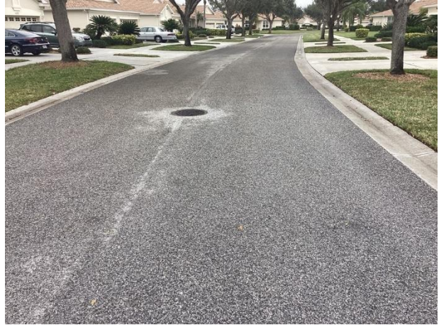
Pavement overview – Magnolia Circle
