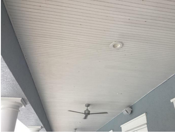
Vinyl soffit overview
