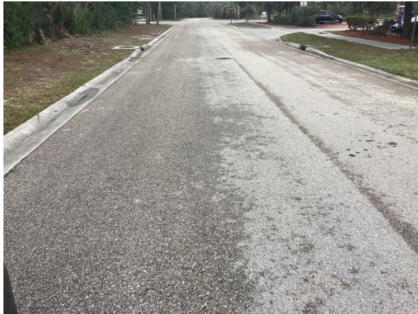
Pavement overview – Sycamore Drive
