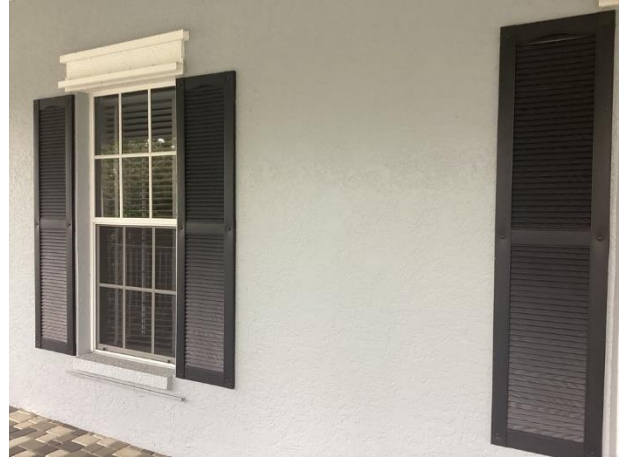
Stucco wall finishes
