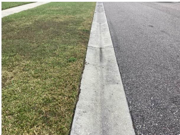
Concrete curb and gutter
