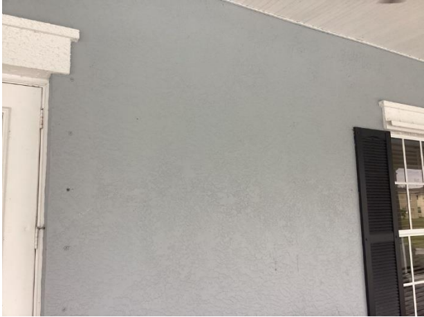
Stucco wall finishes
